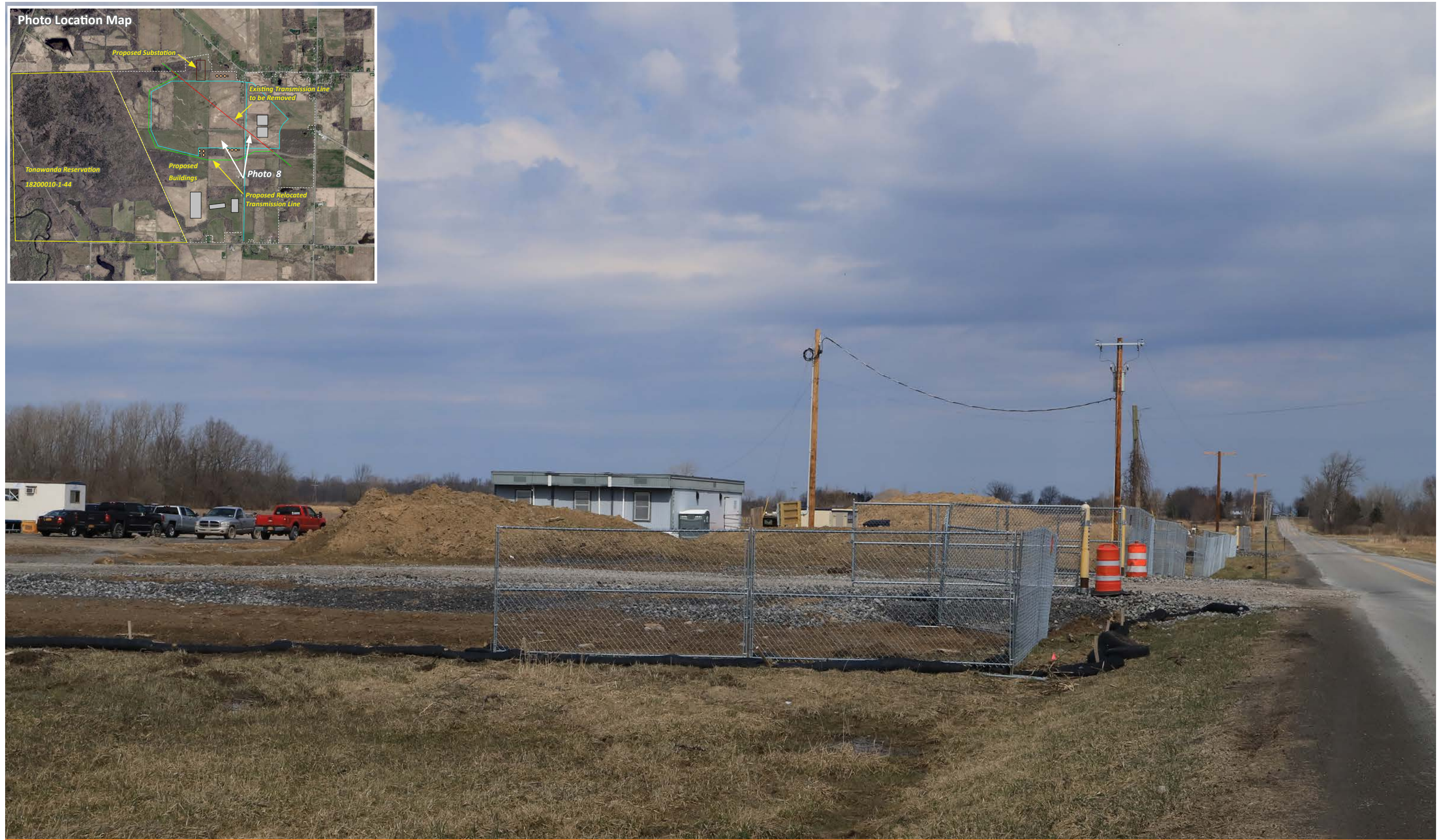
PHOTO 8 CROSBY ROAD - EXISTING CONDITION
