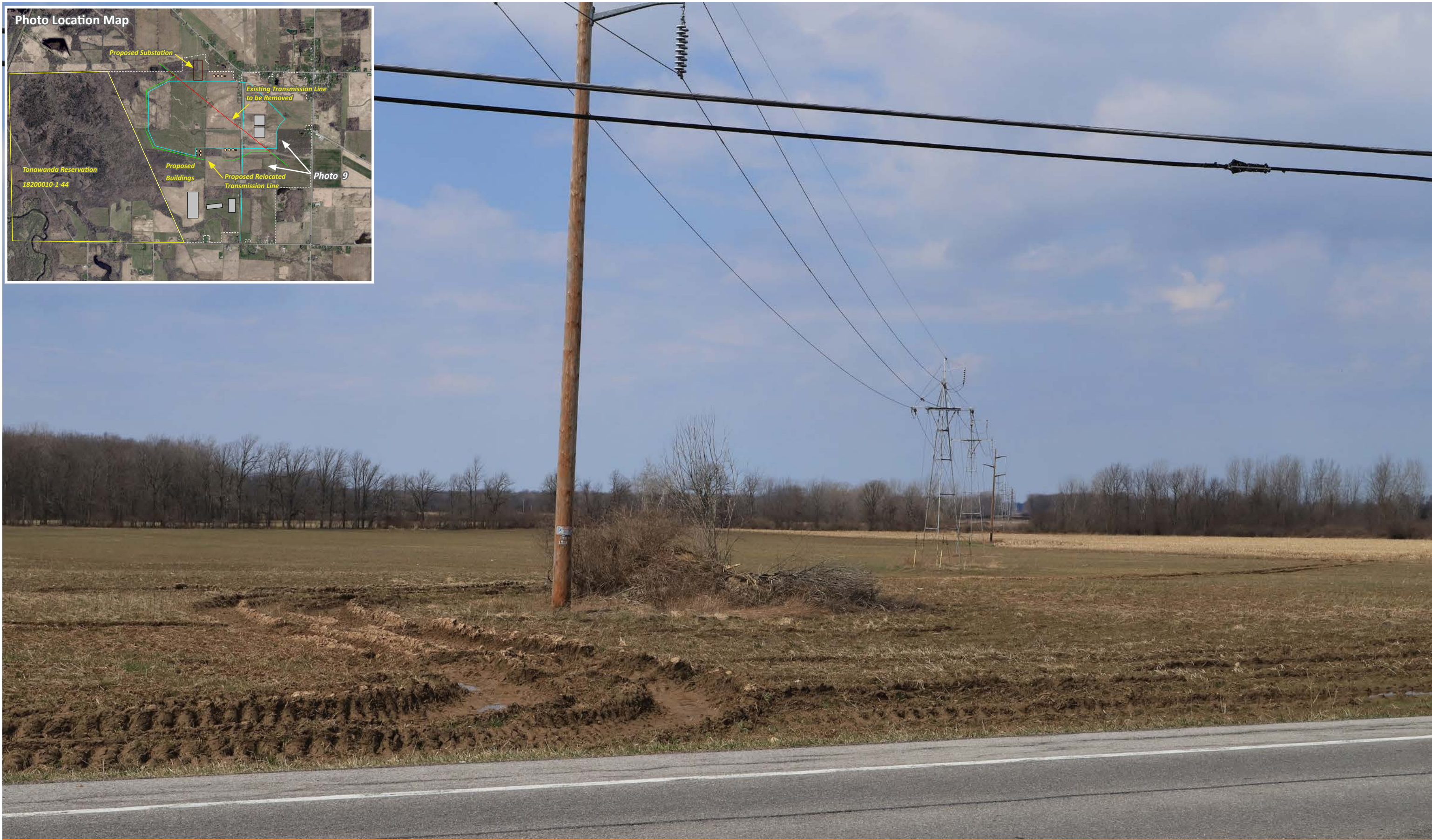
PHOTO 9 ALLEGHENY ROAD - EXISTING CONDITION
