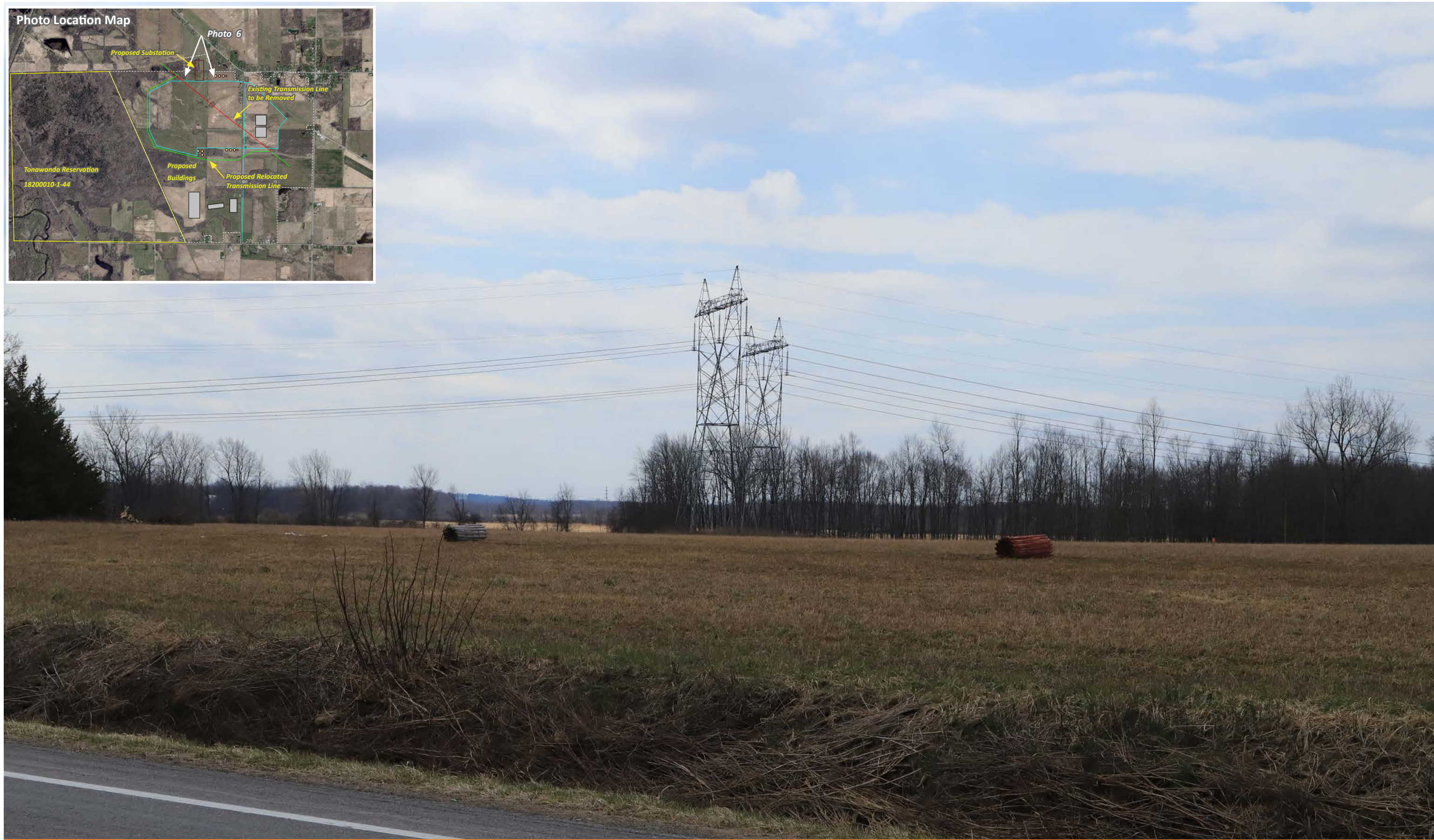
PHOTO 6 LEWISTON ROAD - EXISTING CONDITION
