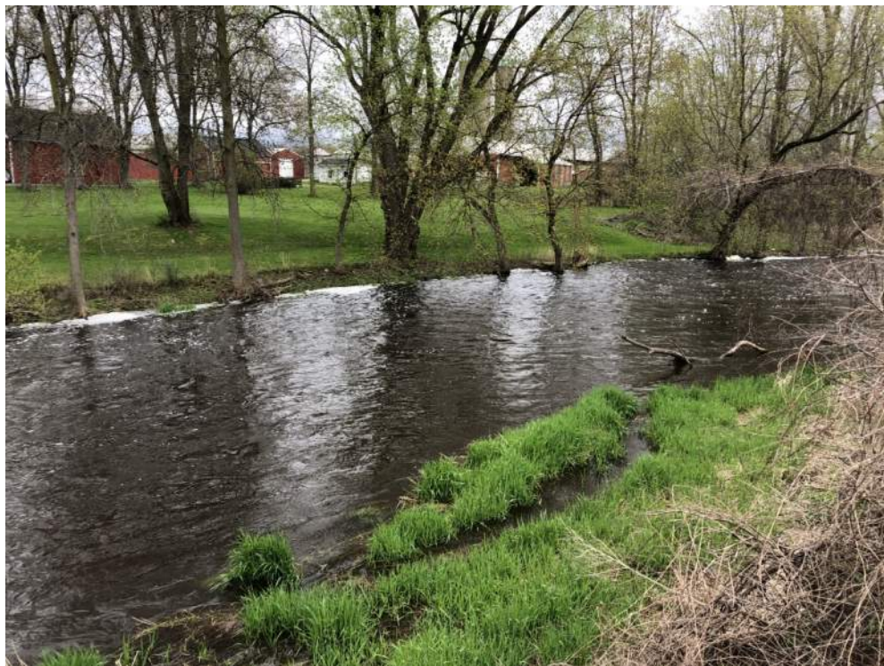
Photo 6: Looking upstream from Maple Ridge Road bridge.
