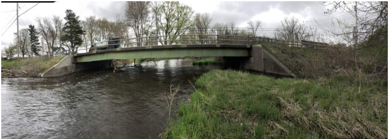
Photo 8: Looking upstream at Maple Ridge Road bridge.
