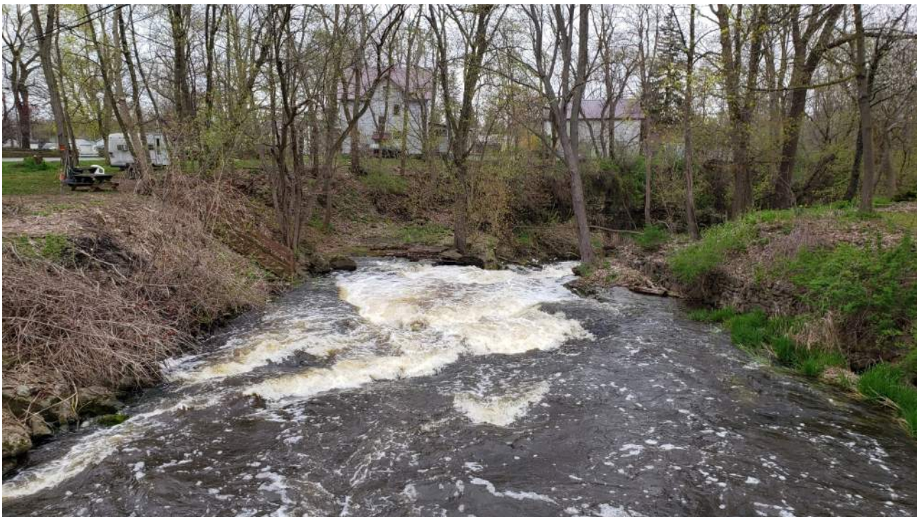
Photo 4: Looking downstream from Main Street bridge.
