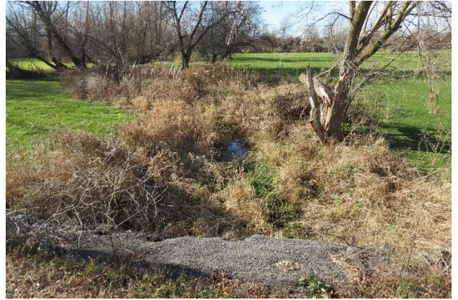
Point 800 – Knowlesville Rd Stream Crossing
