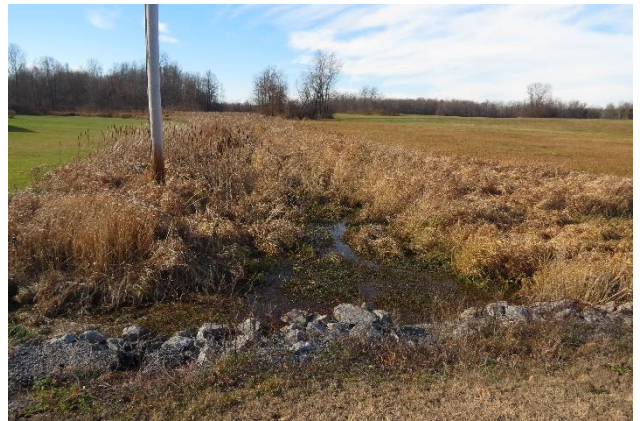
Point 801 – Knowlesville Rd stream crossing
