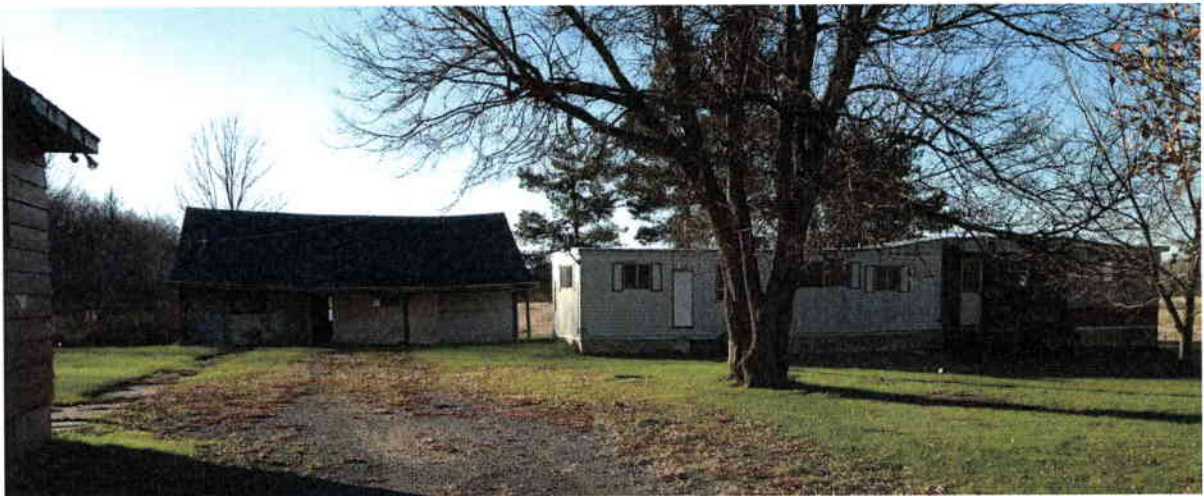
Photo 4. View facing west at the circa 1960 barn / garage and unoccupied trailer associated with the residence at 8420 Crosby Road which is partially visible at the left.
