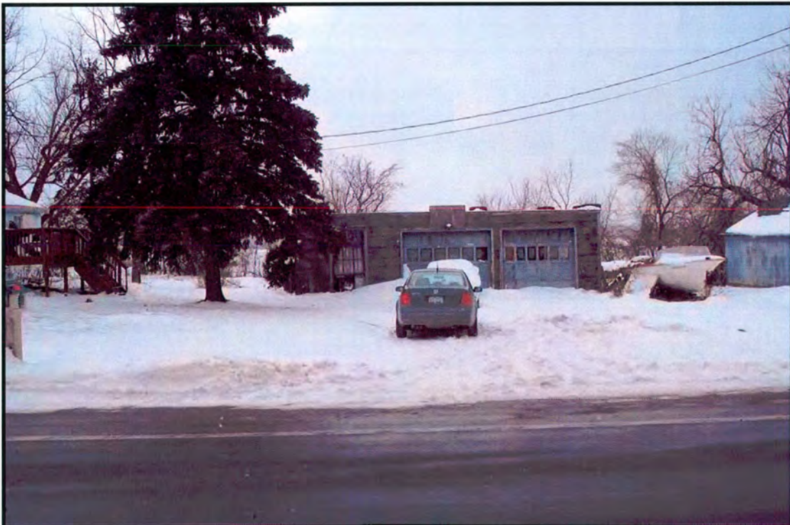
Photo 28. Facing southwest from Lewiston Rd showing garage at 1138 Lewiston Rd (B: 12). This garage is adjacent to the project area and 50+ years old.
