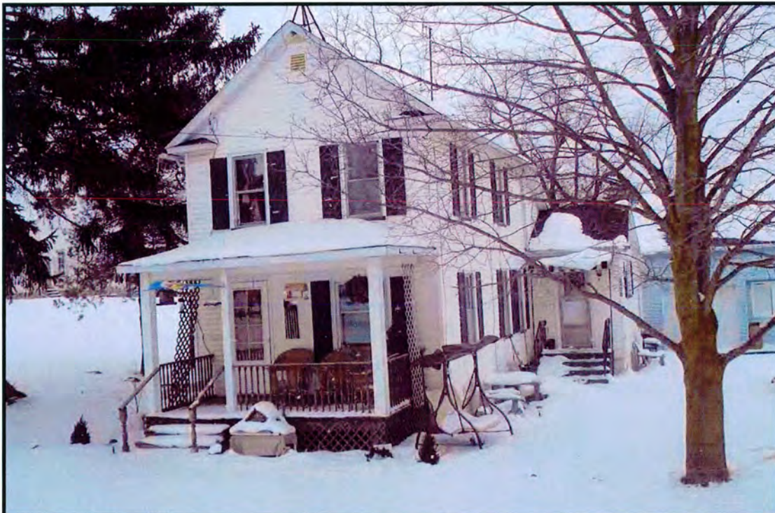
Photo 52. Facing west from Alleghany Rd showing house #6578 (B: 11). This house is adjacent to the project area and 50+ years old.
