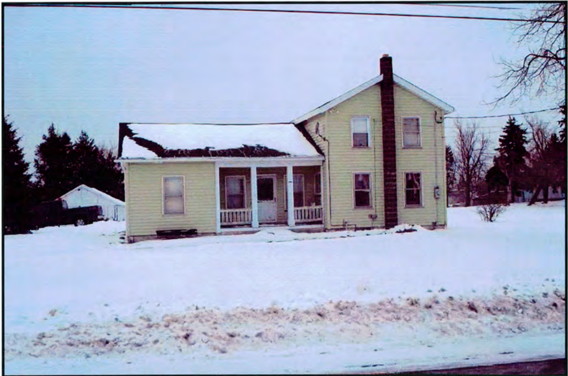
Photo 25. Facing west from Crosby Rd showing house #6568 (B: 12). This house is adjacent to the project area and 50+ years old.
