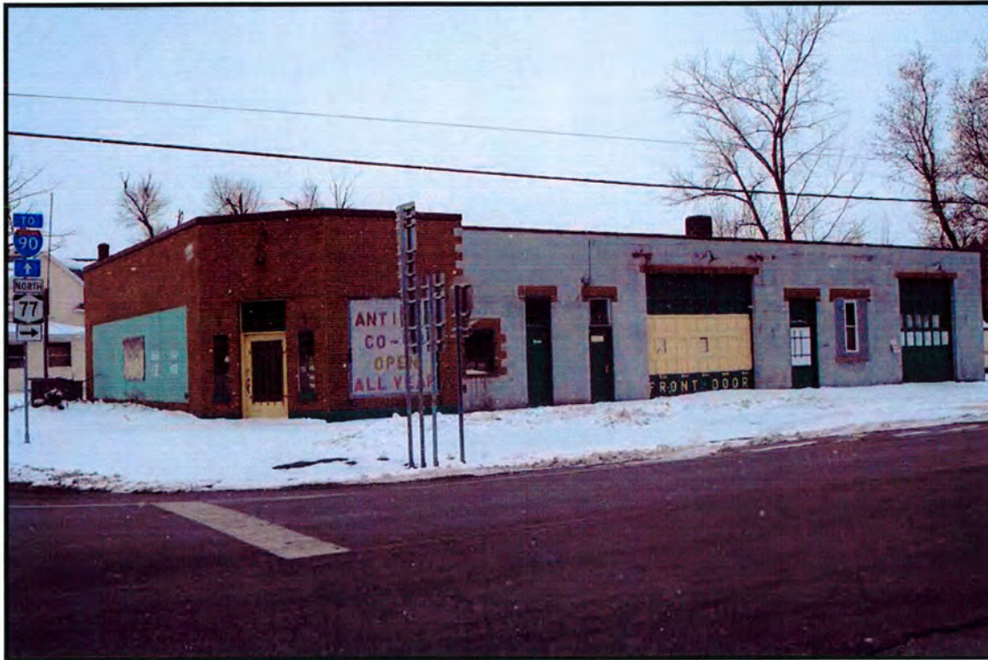
Photo 43. Facing southwest from intersection of Lewiston Rd and Allegheny Rd showing masonry building 50+ years old adjacent to the project area (B: 11). No street address posted.
