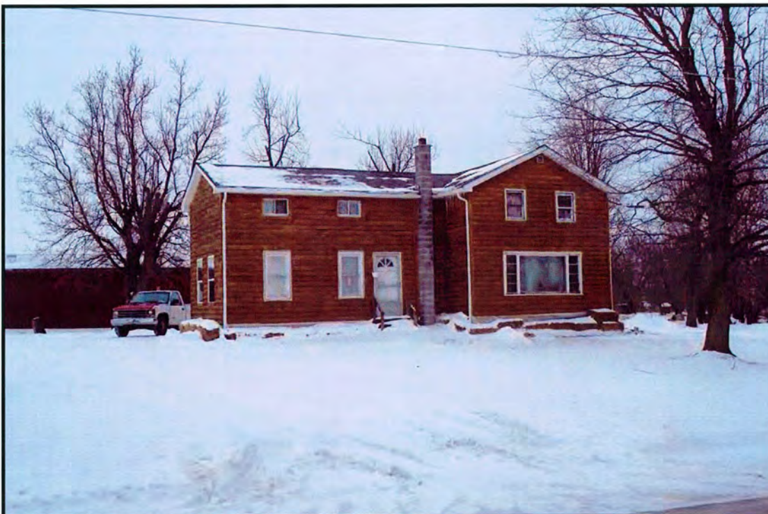
Photo 4. Facing south from Judge Rd showing house #1276 (B: 2). This house is adjacent to the project area and 50+ years old.
