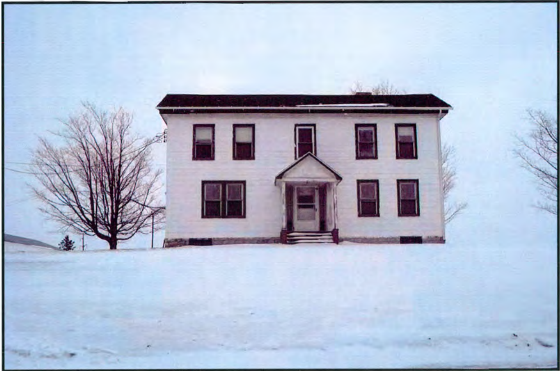
Photo 65. Facing east from Alleghany Rd showing house #6889 (B: 2). This house is adjacent to the project area and 50+ years old.
