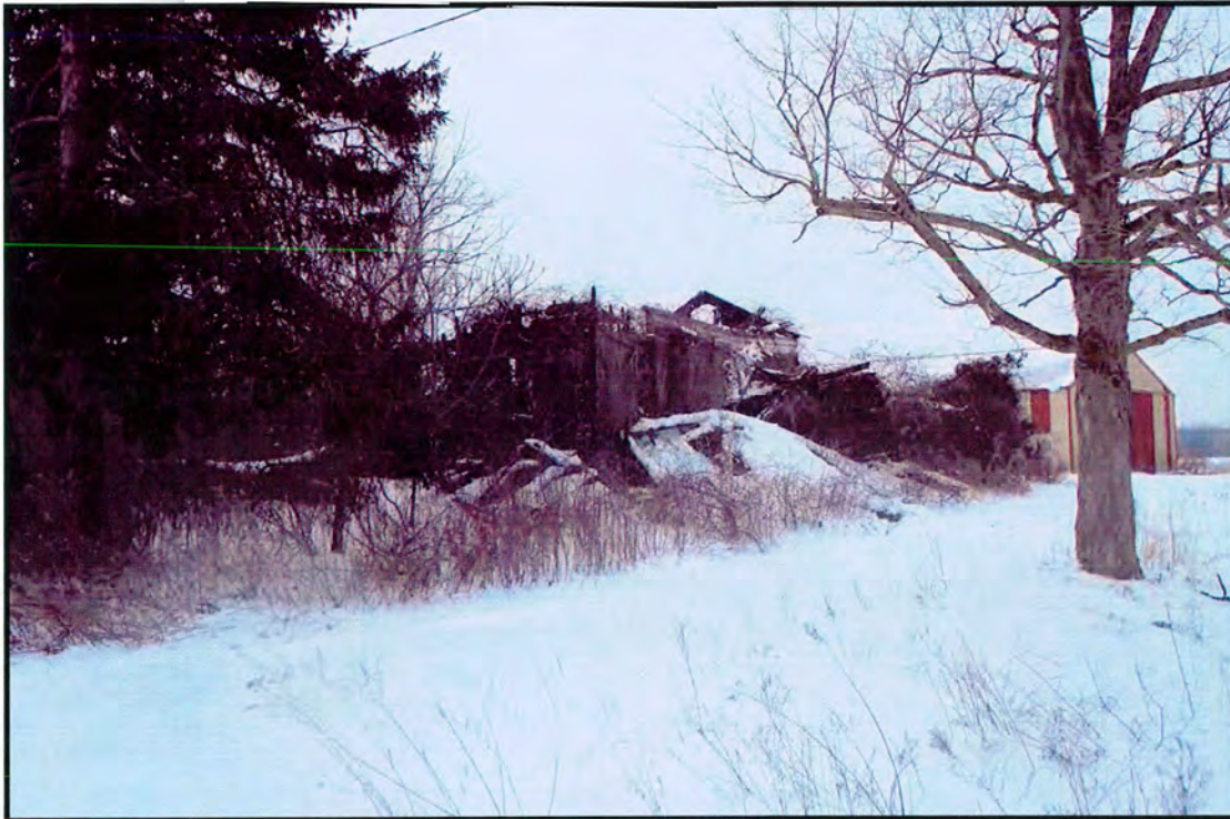
Photo 19. Facing southwest from Crosby Rd showing collapsed house 50+ years old (B: 6). This house is within the project area, and is indicated on the 1904 historic map as the J. Potter estate (Figure 7).
