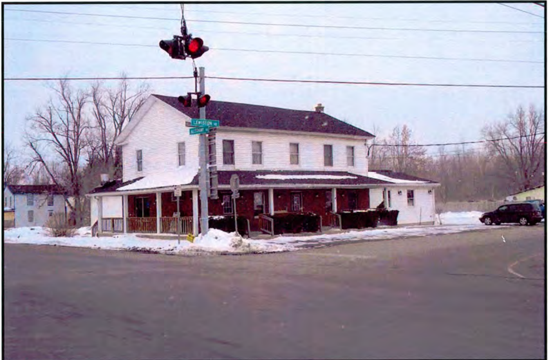
Photo 42. Facing northeast from intersection of Lewiston Rd and Alleghany Rd showing Alabama Hotel (B: 11). This building is adjacent to the project area and 50+ years old. No street address posted.
