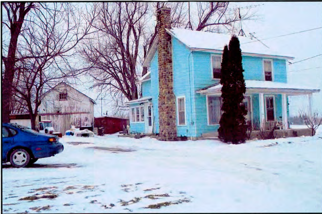
Photo 63. Facing northwest from Alleghany Rd showing house #6686 and barn 50+ years old (B: 8). The house and barn are adjacent to the project area.
