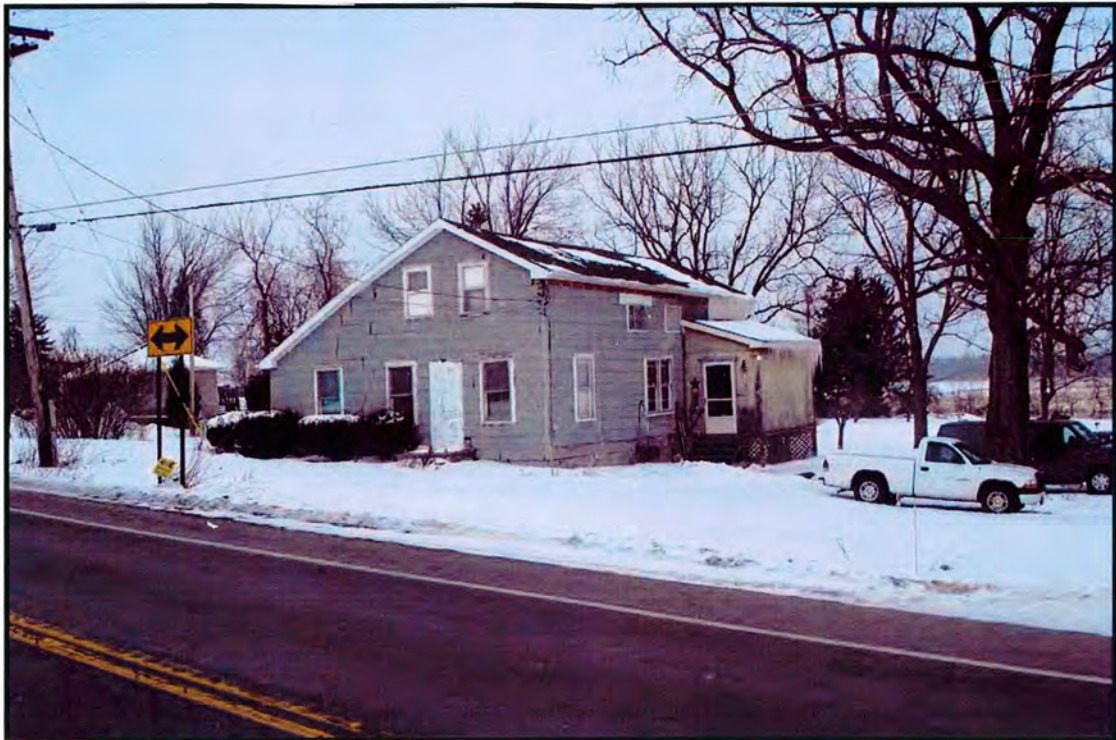
Photo 29. Facing north-northwest from Lewiston Rd showing house #1147 (B: 12). This house is adjacent to the project area and 50+ years old.
