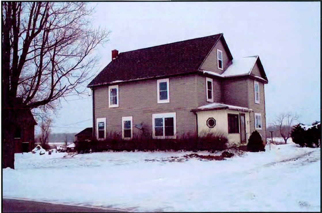
Photo 6. Facing north-northwest from Judge Rd showing house 50+ years old (B: 2). This house is within the project area, and is indicated on the 1904 historic map as the Hodgins residence (Figure 7). No street address posted.
