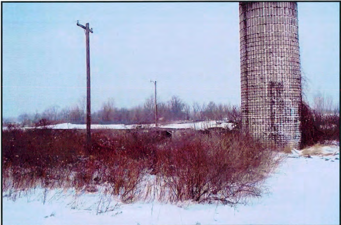
Photo 14. Facing north from Judge Rd showing silo and collapsed barn 50+ years old (B: 3). The barn and silo are within the project area. On the 1904 historic map, the barn is located on the W. Pickworth property (Figure 7).
