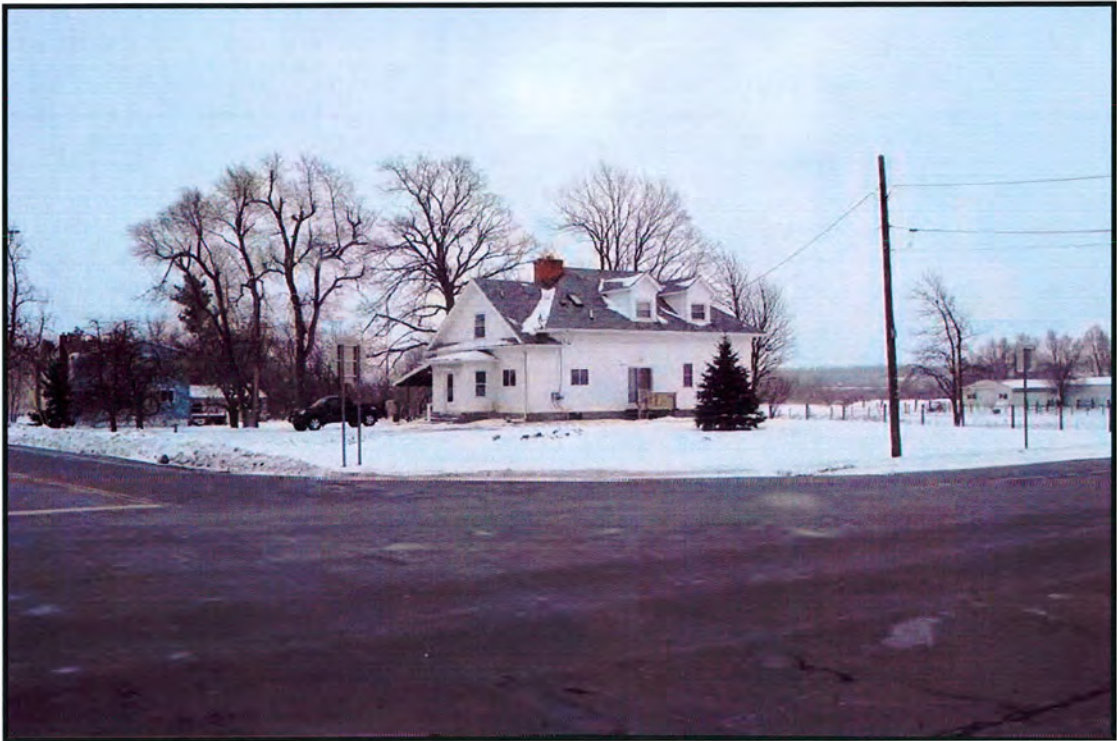
Photo 1. Facing southeast from intersection of Alleghany Rd and Judge Rd showing house #1358 (see Attachment B: 2). This house is adjacent to the project area and 50+ years old.
