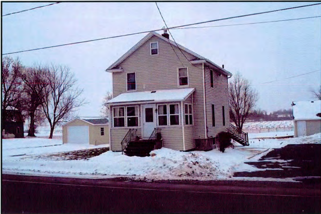
Photo 48. Facing west from Alleghany Rd showing house #6560 (B: 11). This house is adjacent to the project area and 50+ years old.
