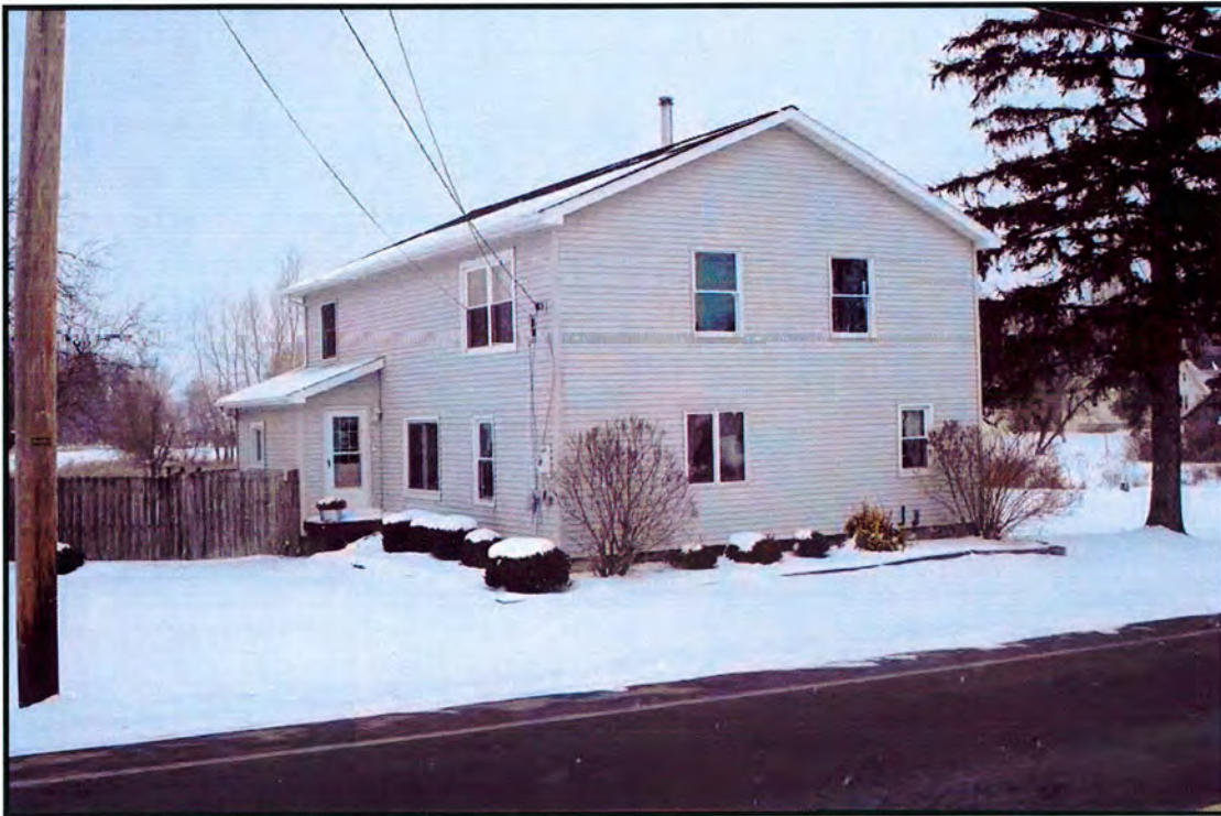
Photo 39. Facing north-northeast from Lewiston Rd showing house 50+ years old (B: 11). This house is adjacent to the project area. No street address posted.
