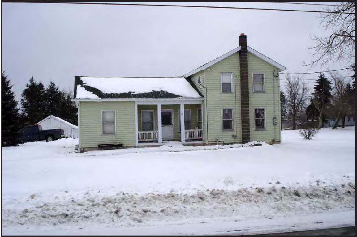
Photo 25. Facing west from Crosby Rd showing house #6568 (B: 12). This house is adjacent to the project area and 50+ years old.
