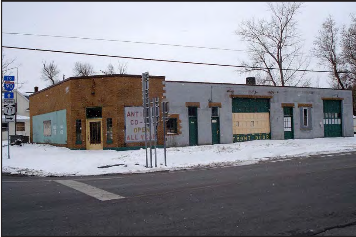
Photo 43. Facing southwest from intersection of Lewiston Rd and Alleghany Rd showing masonry building 50+ years old adjacent to the project area (B: 11). No street address posted.
