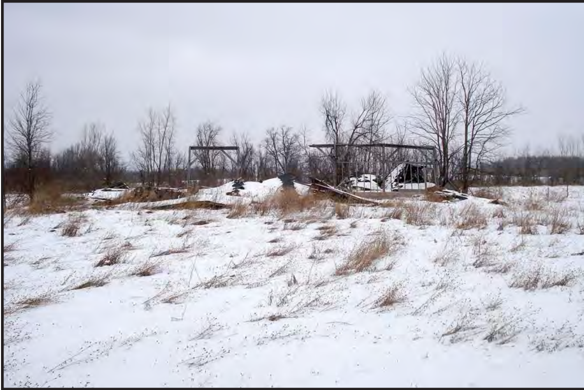
Photo 15. Facing north from Judge Rd showing collapsed barn 50+ years old (B: 3). This barn is within the project area. On the 1904 historic map, the barn is located on the W. Pickworth property (Figure 7).
