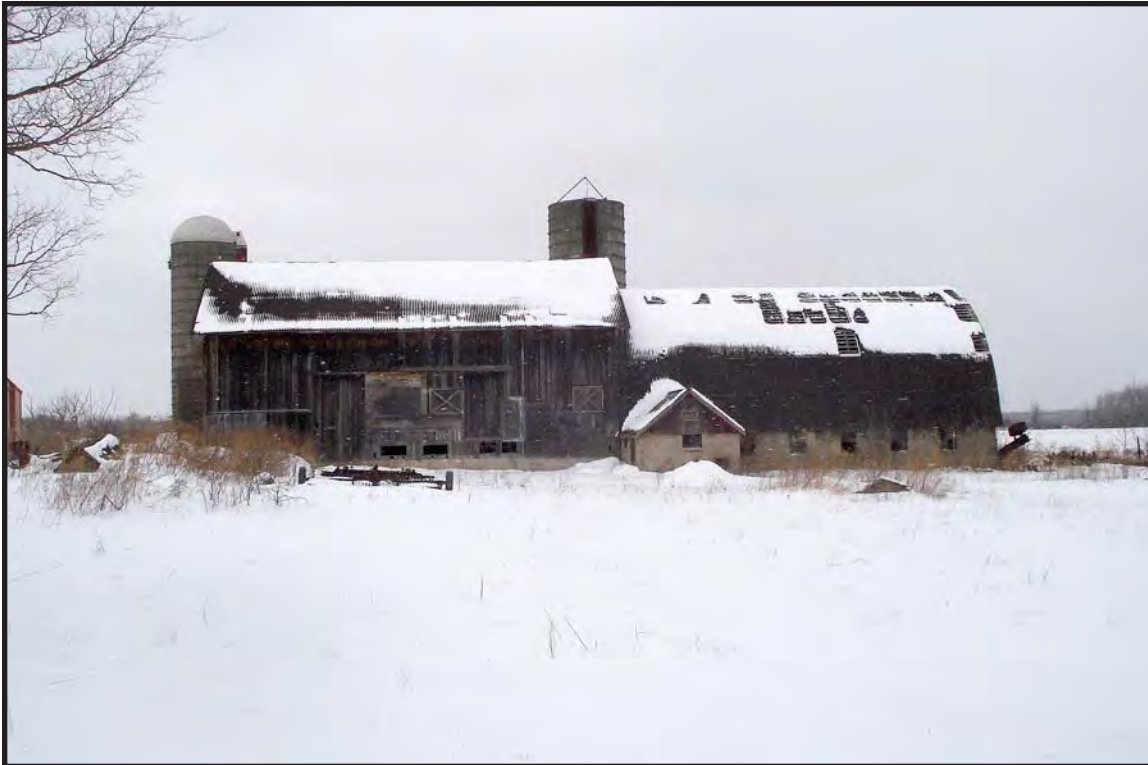
Photo 20. Facing west from Crosby Rd showing barn complex and silos 50+ years old (B: 6). The barn complex is within the project area. On the 1904 historic map, the barn complex is located on the J. Potter estate (Figure 7).
