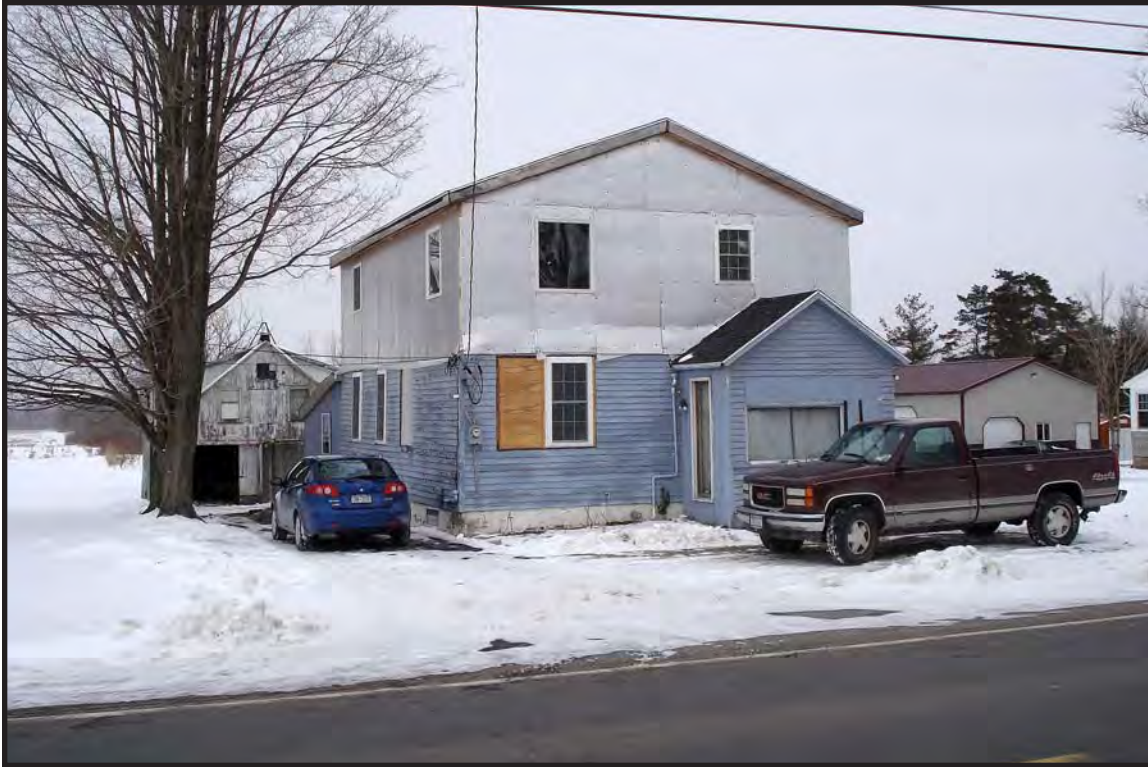
Photo 35. Facing north-northeast from Lewiston Rd showing house #1261 and garage 50+ years old (B: 11). The house and garage are adjacent to the project area.
