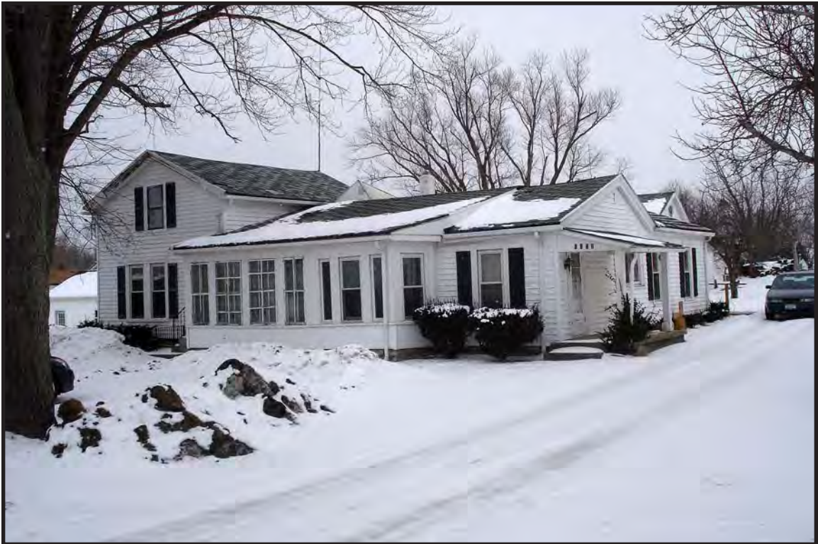
Photo 45. Facing east from Alleghany Rd showing house #6553 (B: 11). This house is adjacent to the project area and 50+ years old.
