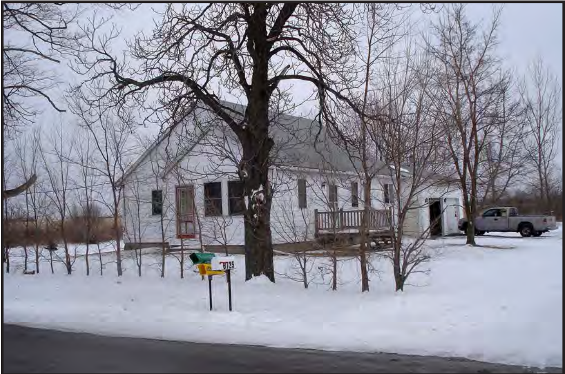
Photo 22. Facing northeast from Crosby Rd showing house #6725 (B: 9). This house is within the project area and appears to be 50+ years old. The W. Donnan and S. Hoover residence is indicated at this location on the 1866 and 1904 historic maps (Figures 3 and 7).
