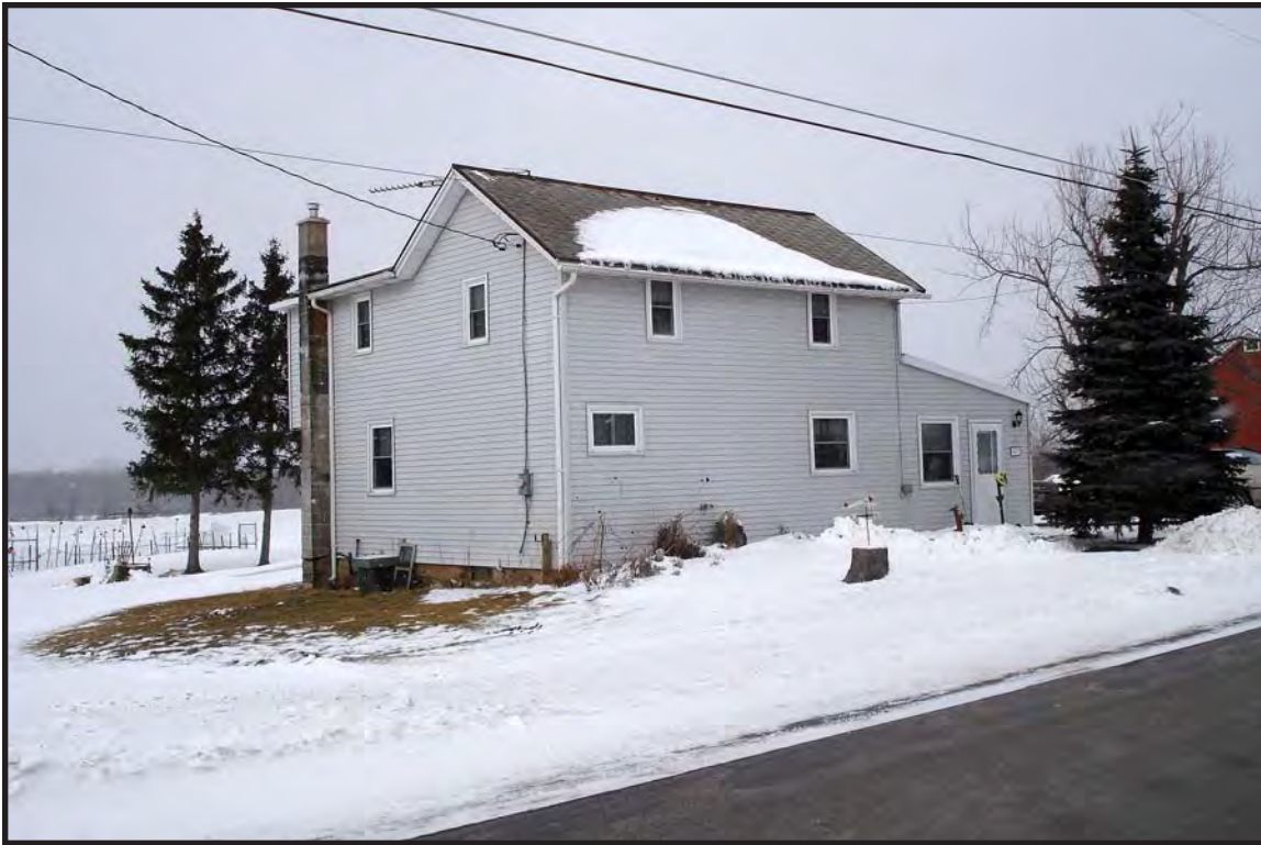
Photo 23. Facing northwest from Crosby Rd showing house #6590 (B: 12). This house is adjacent to the project area and 50+ years old.
