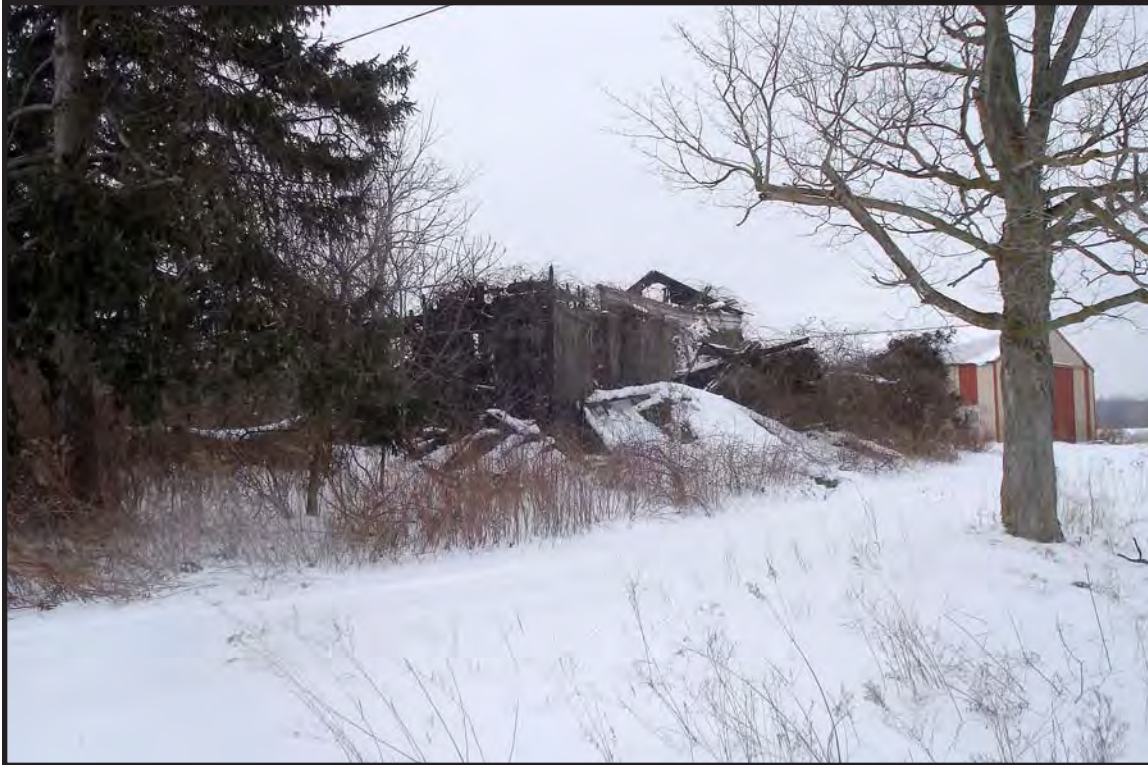
Photo 19. Facing southwest from Crosby Rd showing collapsed house 50+ years old (B: 6). This house is within the project area, and is indicated on the 1904 historic map as the J. Potter estate (Figure 7).
