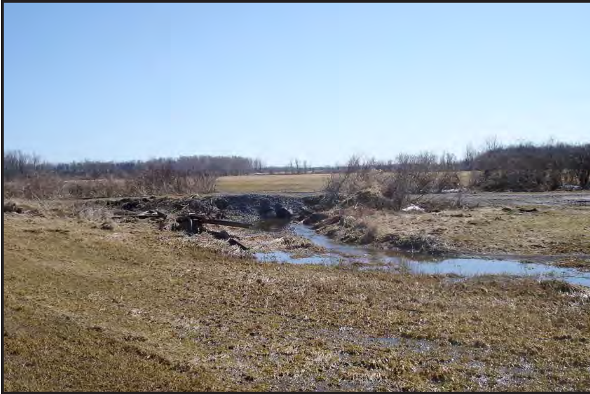
Photo 99. Facing south showing culvert along Patterson Rd (abandoned) (B: 9).
