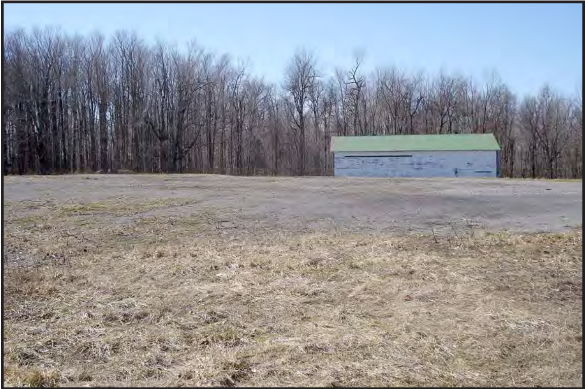
Photo 66. Facing west near entrance of John White Wildlife Management Area (JWWMA) showing barn 50+ years old (B: 2). This barn is within the project area, and is located on the B. Norton, D. Norton and A. P. Norton property on the historic maps (Figures 3, 5 and 7).
