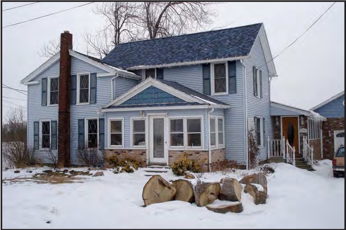
Photo 2. Facing north from Judge Rd showing house #1339 (B: 2). This house is adjacent to the project area and 50+ years old.
