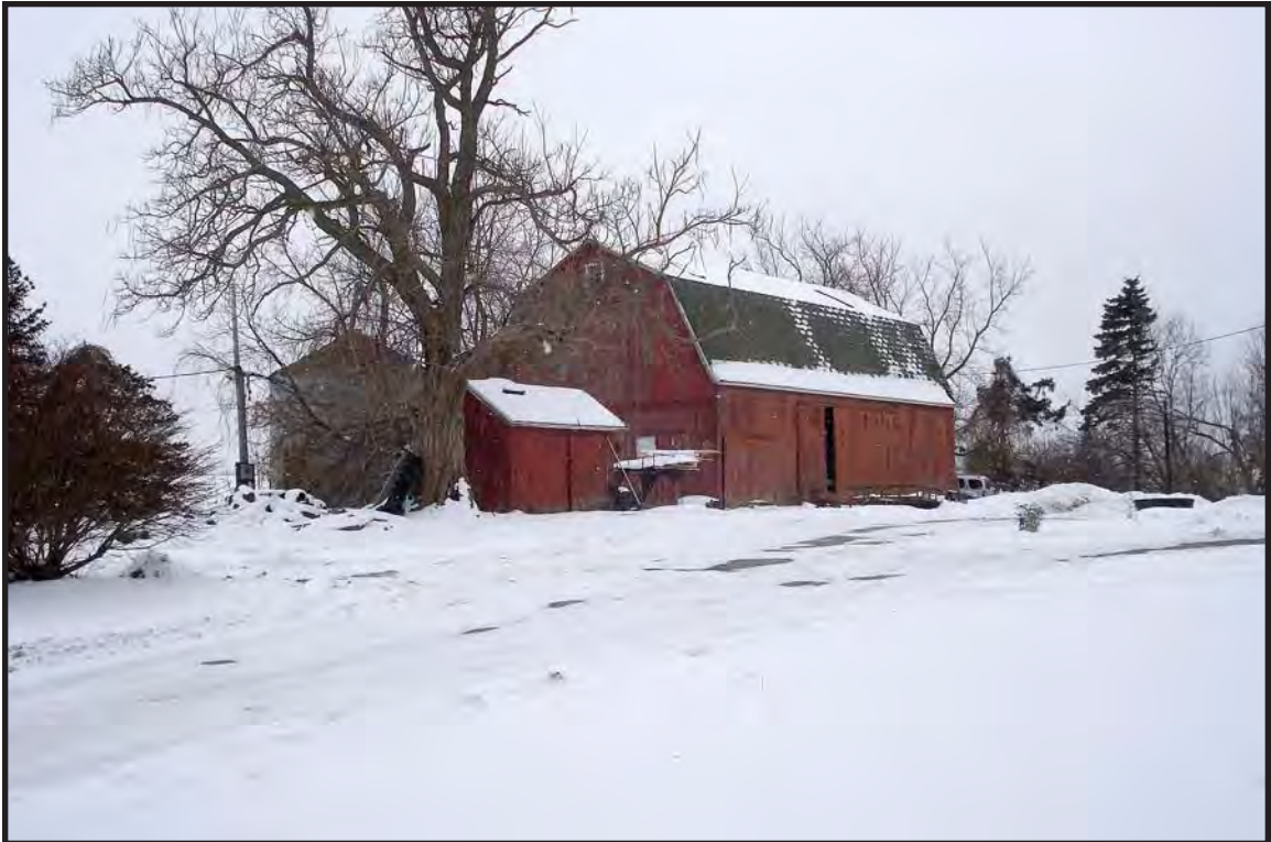
Photo 62. Facing southwest from Alleghany Rd showing barn complex at 6604 Alleghany Rd (B: 11). The barn complex is within the project area and 50+ years old. On the 1904 historic map, the barn is located on the Norton property (Figure 8).
