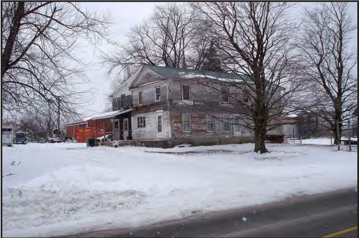
Photo 10. Facing southwest from Judge Rd showing house #1120 (B: 3). This house is adjacent to the project area and 50+ years old.
