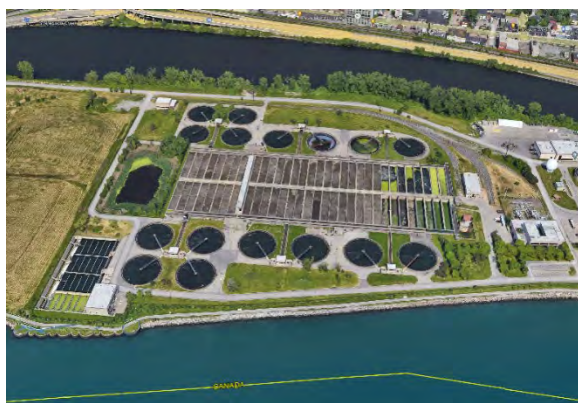
Figure 1 Bird Island WWTF
