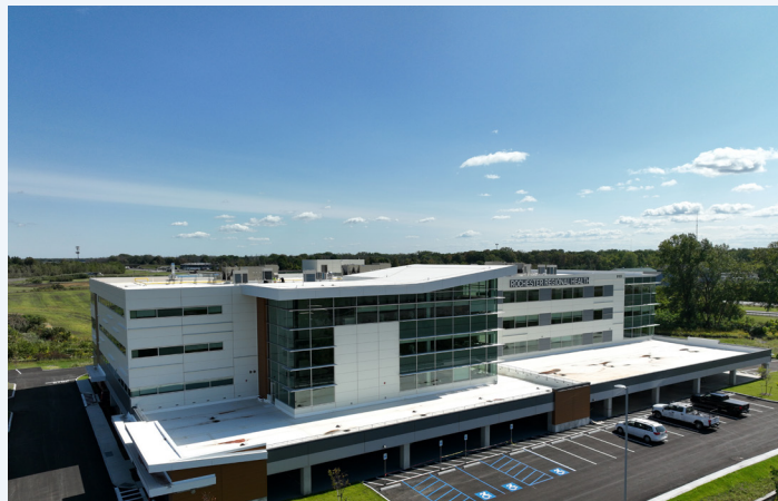
In 2023, Rochester Regional Health completed the four-story Batavia Medical Campus, a destination campus with more than a dozen specialty areas. The GCFC supported this healthcare project with tax-exempt bonding.
