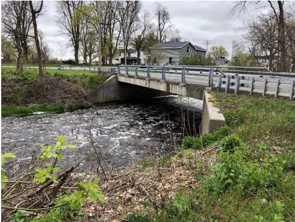
Photo 3: Looking upstream from left bank at Main Street bridge.
