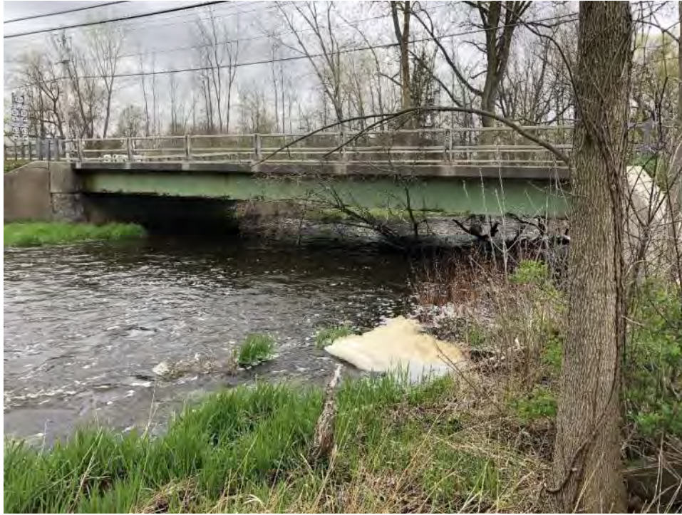
Photo 7: Looking downstream from right bank at Maple Ridge Road bridge.
