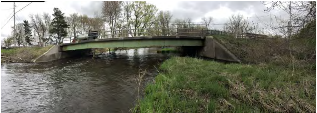
Photo 8: Looking upstream at Maple Ridge Road bridge.
